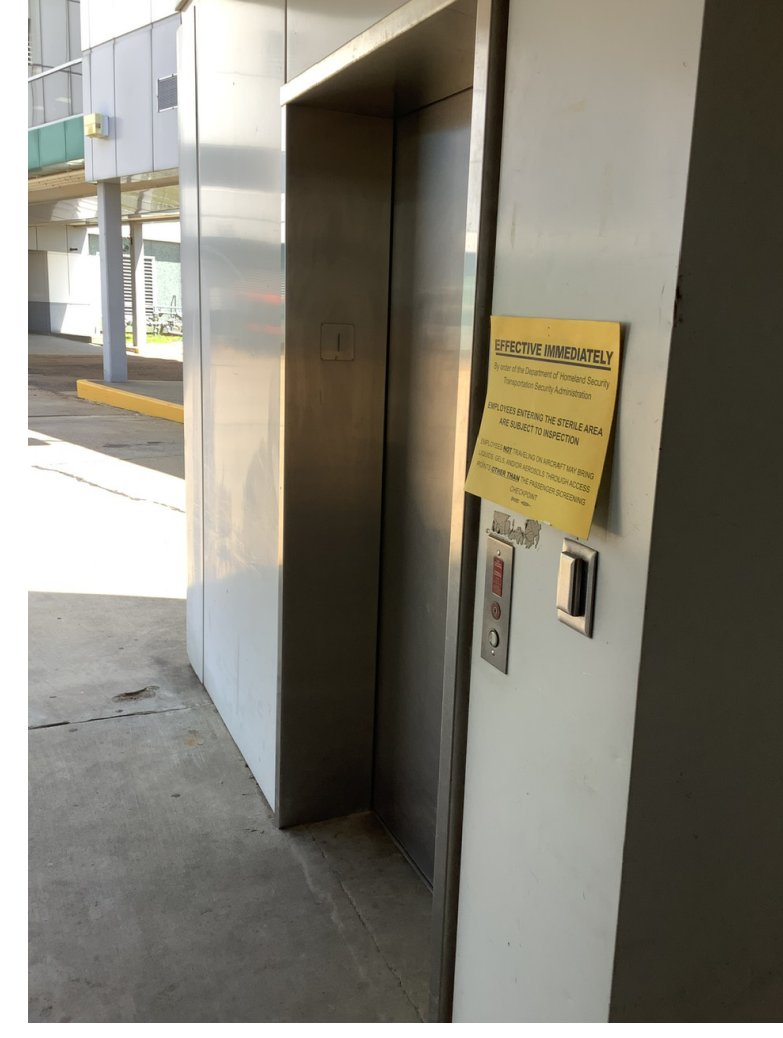
PHOTO #2 - ELEVATOR #4 - EXTERIOR ON 1ST LEVEL
