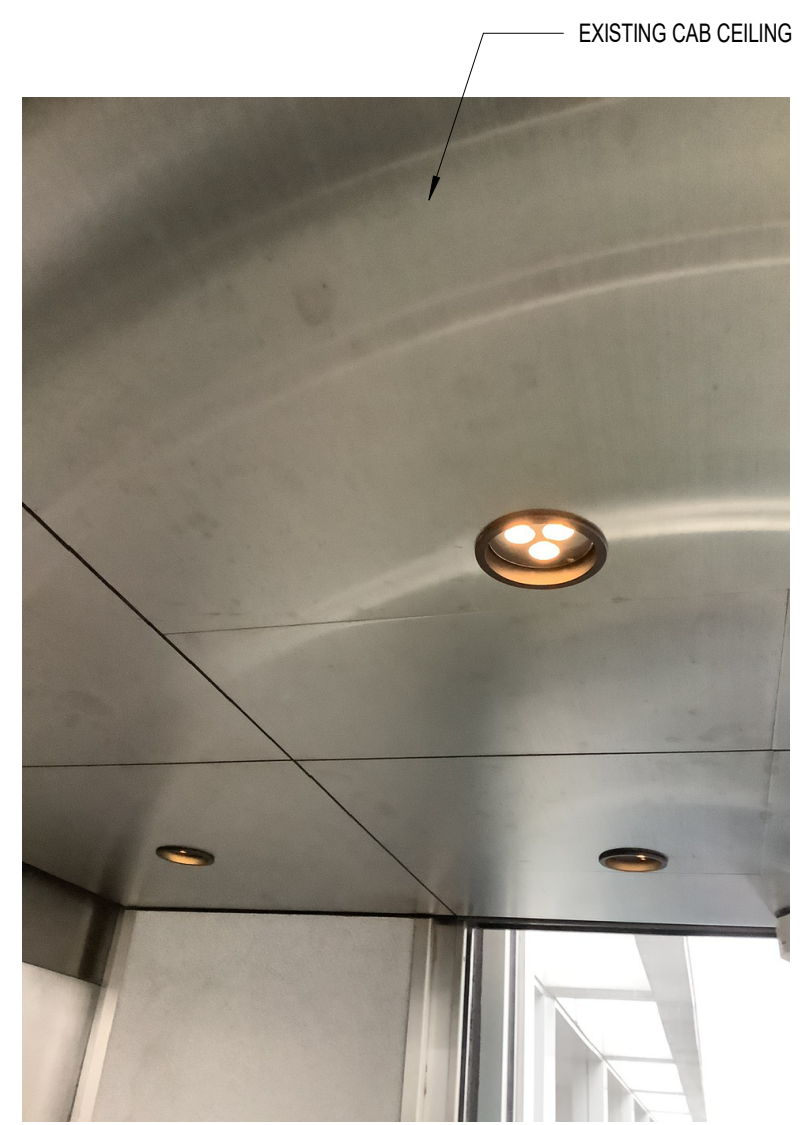
PHOTO #6 - ELEVATOR #3 - EXISTING CABIN CEILING
