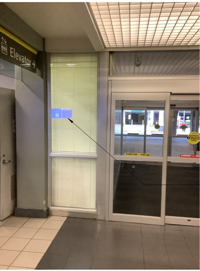
PHOTO #5 - ELEVATOR #3 - LOBBY
