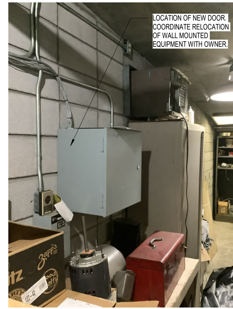
PHOTO #7 - ELEVATOR #4 - STORAGE AREA
