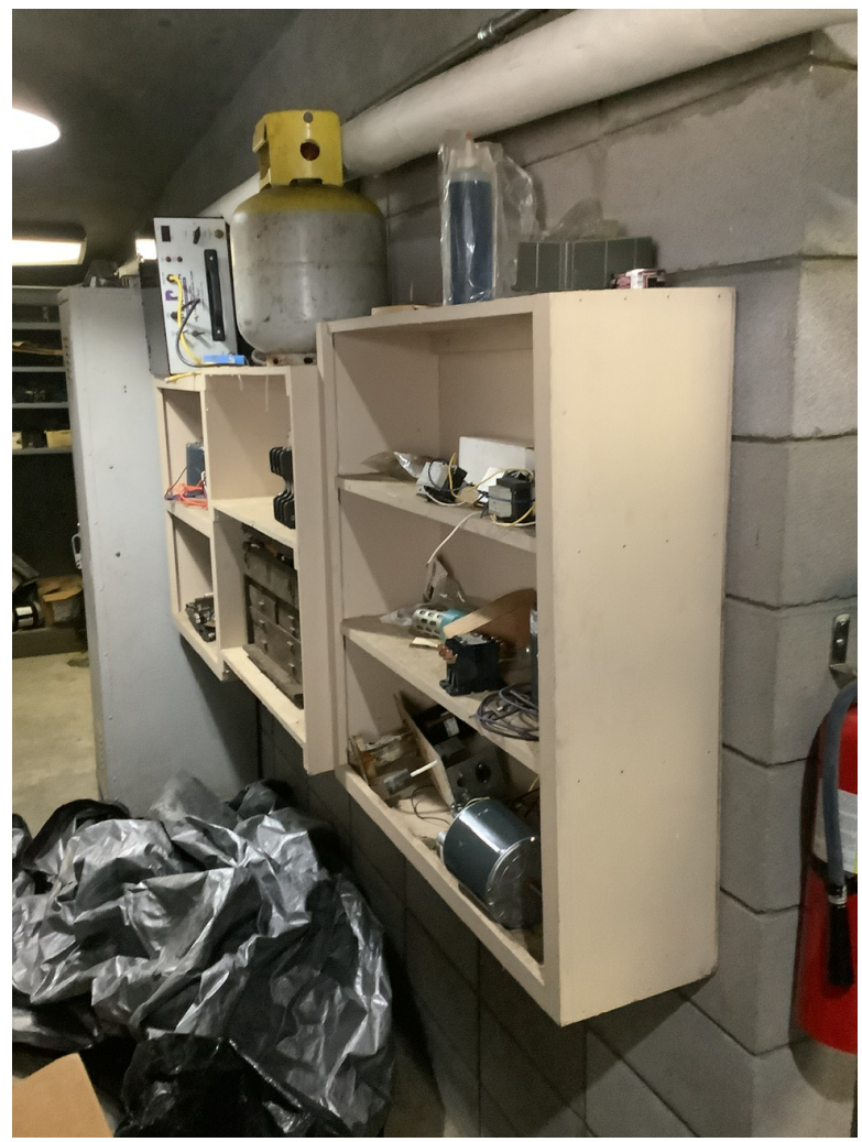
PHOTO #9 - ELEVATOR #4 - STORAGE AREA
