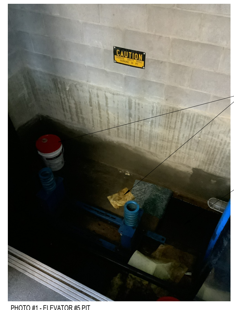
PHOTO #1 - ELEVATOR #5 PIT
