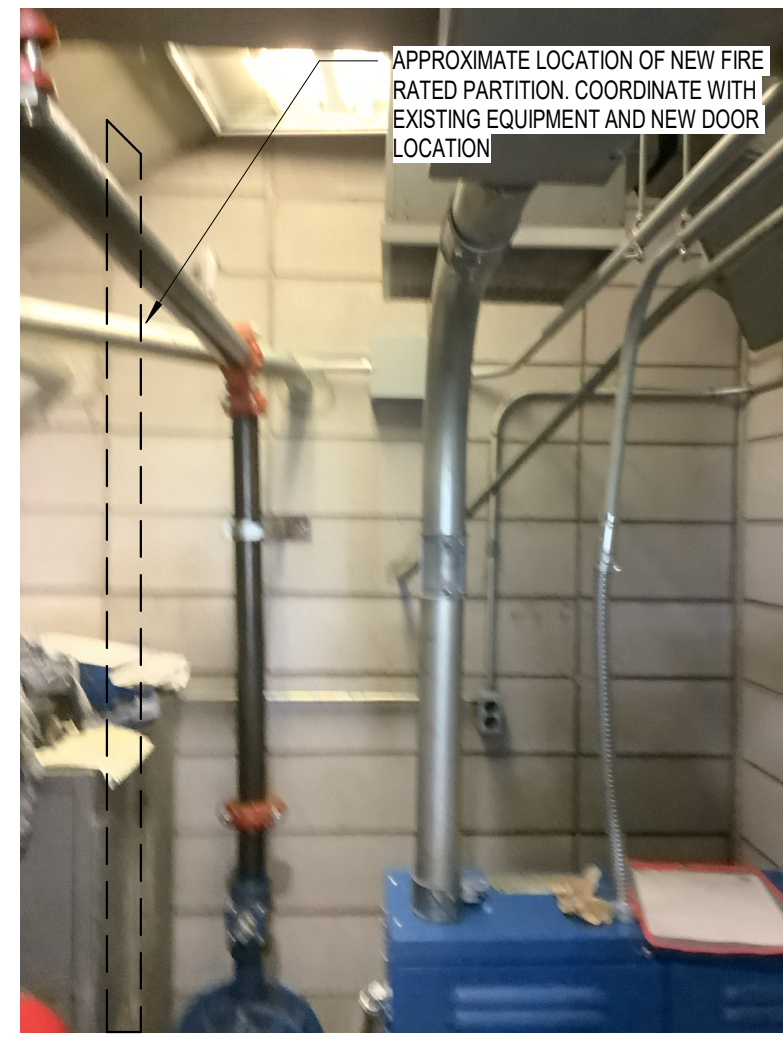
PHOTO #8 - ELEVATOR #4 - MACHINE AREA
